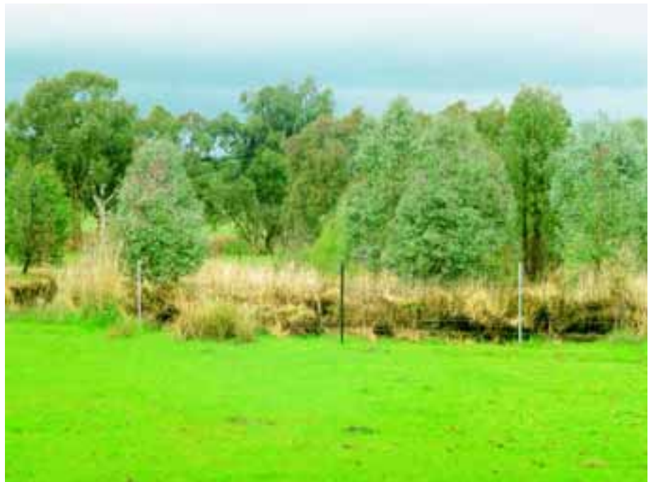
After. A rock chute has been built and extensive revegetation works undertaken. The gully now delivers clean water downstream.
