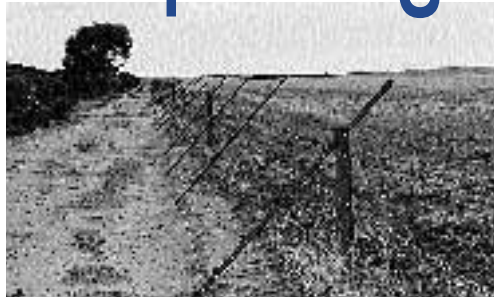
Ten wire sloping fence has four live and six earth wires. Materials costs were $1,600/km.
